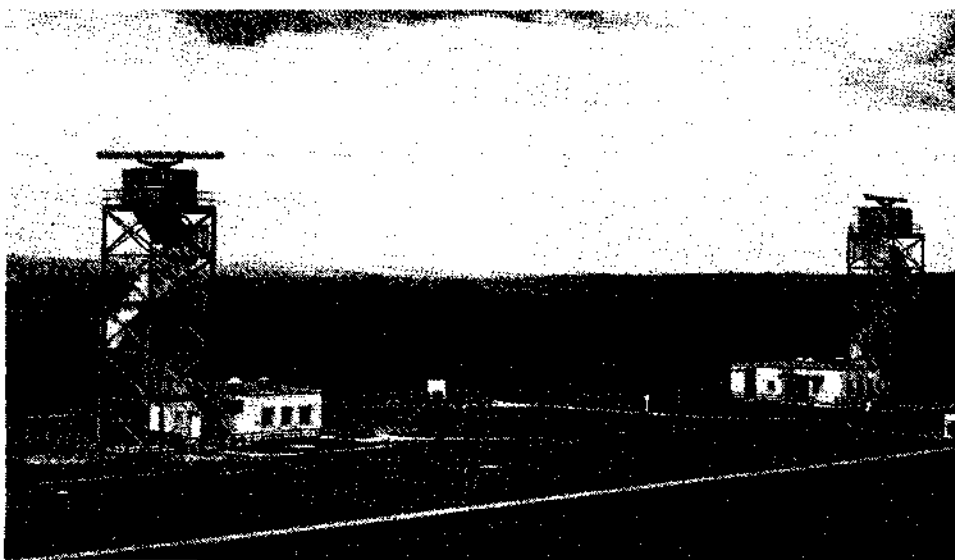
The Cossor SSR installation at Burrington, Devon
