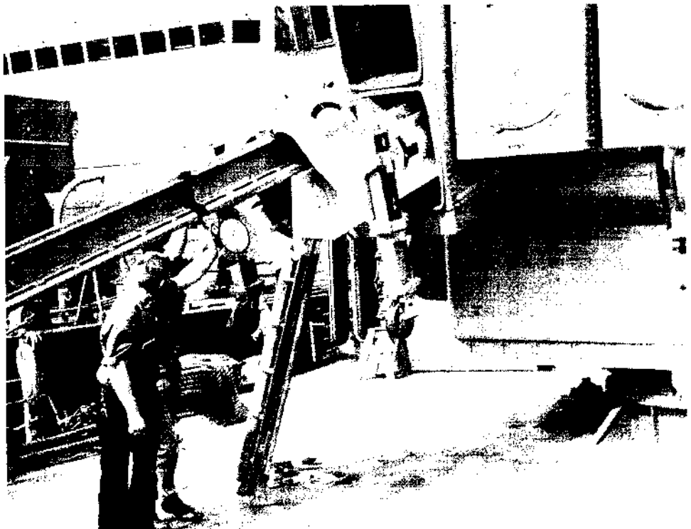
Loading of Standard (RIM-66A) MR missile into its launcher container
