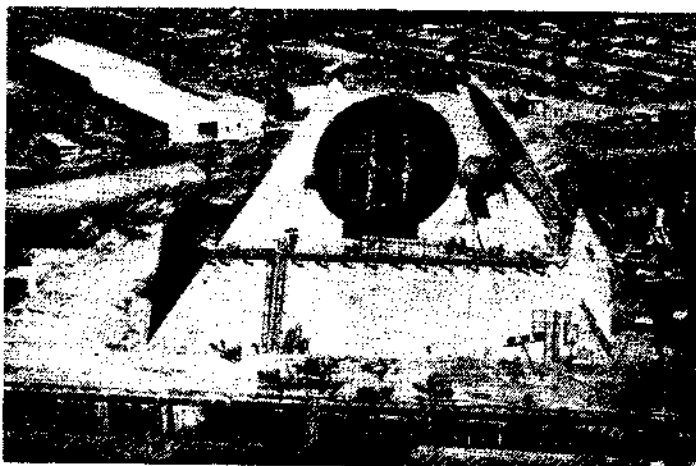
Missile Site Radar (SR) and Perimeter Acquisition Radar (PAR) under construction at North Dakota sites. The SR (left) will have phased rays on each of its four sloping faces and will have a detection range of several hundred kilometres on a re-entry vehicle. The PAR building shown on the right is a kind intended to have only one phased array (on its sloping face): PARs proposed for some other sites would have had arrays on more than one face
