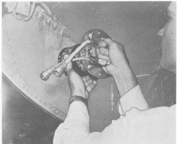
3 INSERTION OF DESTRUCTOR PACKAGE
