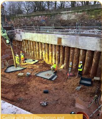
Contig pile wall completion and commencement of basement pile caps
