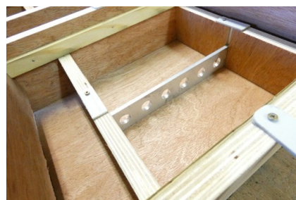
Fig 9 Mounting the Earth Bar
