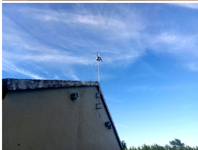
Mounted on the shed gable wall with solar panel facing south
