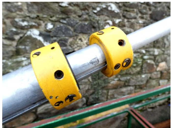
Grooves can be seen here between tubes.
