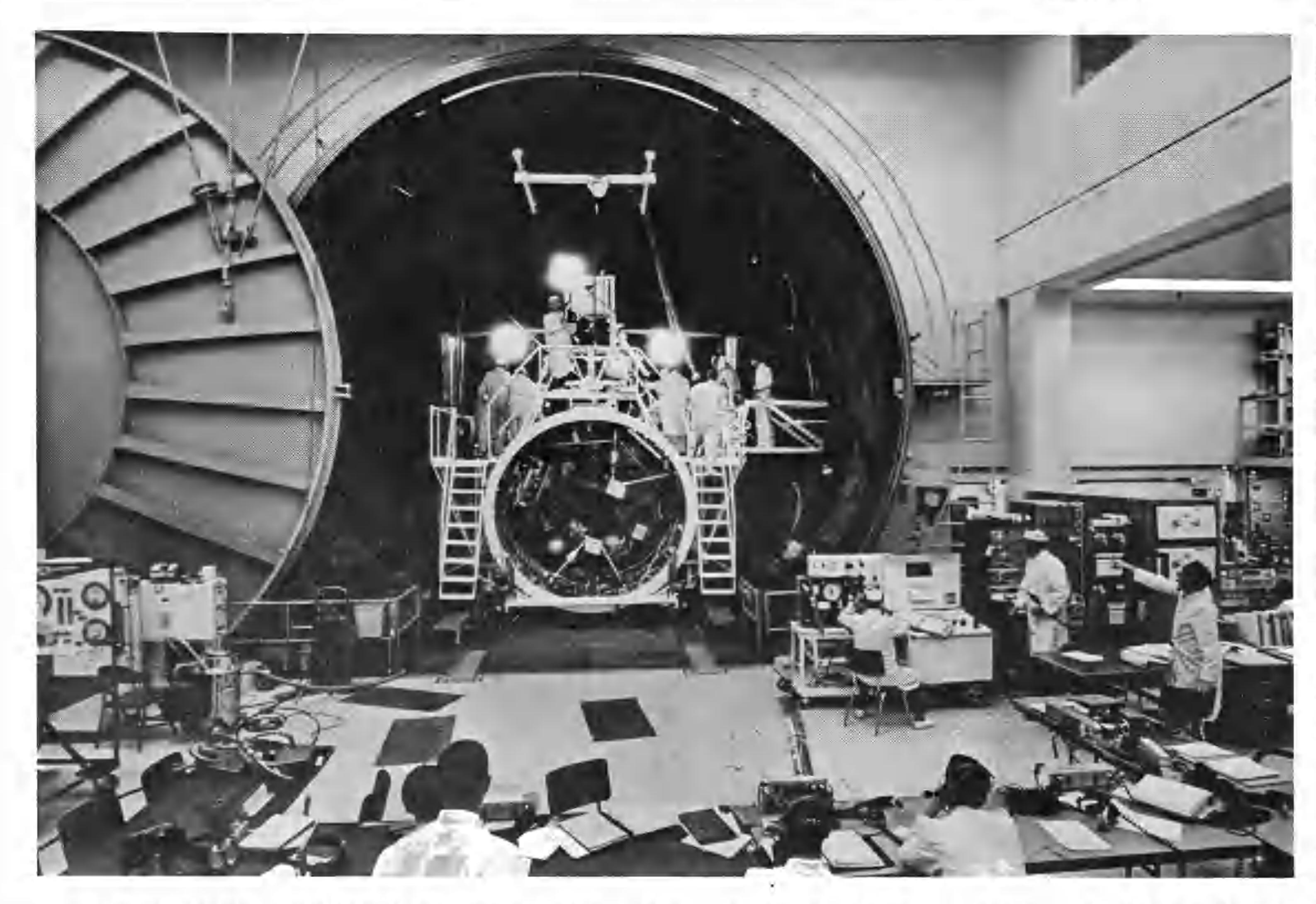
IN 30-FOOT FLIGHT SIMULATION CHAMBER at McDonnell Space Center, Gemini 12 is readied for a simulated mission into the frigid vacuum of outer space. Astronaut training brought both prime and backup crews to McDonnell to "fly" their assigned Gemini on simulated missions. Closing of chamber's sliding door creates a cylinder 30 feet in diameter, 36 feet in length.
