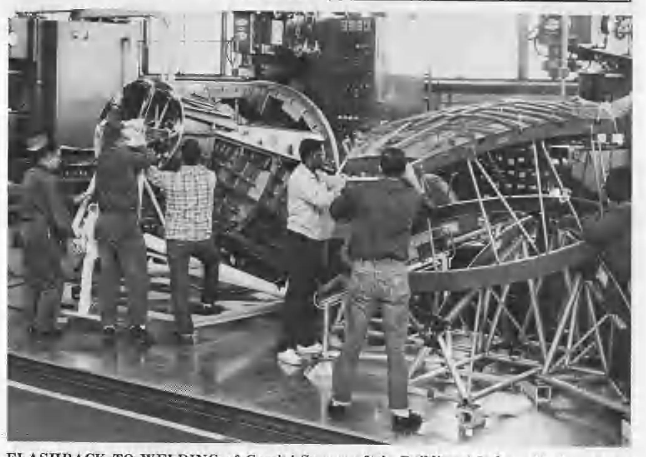
FLASHBACK TO WELDING of Gemini Spacecraft in Building 1 before this important operation was moved to the Space Center. Welders are working on spacecraft's pressurized cabin section which was comprised of 85% welded-titanium assemblies. The welding of titanium to hold tolerances to ±.010 inch was one of the major McDonnell breakthroughs in the Gemini program.
