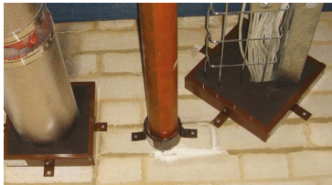
SERVICES THROUGH COLLARS & MULTI PURPOSE BOXES
