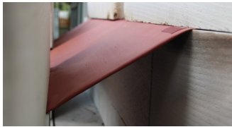
SEALED CAVITY TRAY
