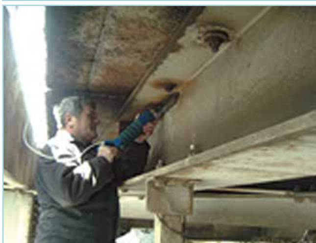
UIT of welded crack (1 m) in Podil railway bridge (Kyiv, Ukraine; without stopping of on-going traffic)
