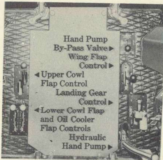
Fig. 10 — Hydraulic Control Panel Looking Aft
