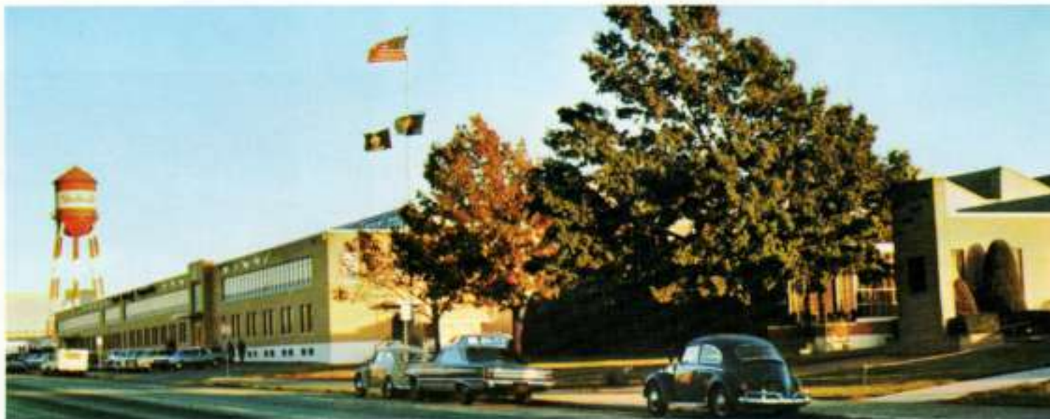
Plant I administration building.
