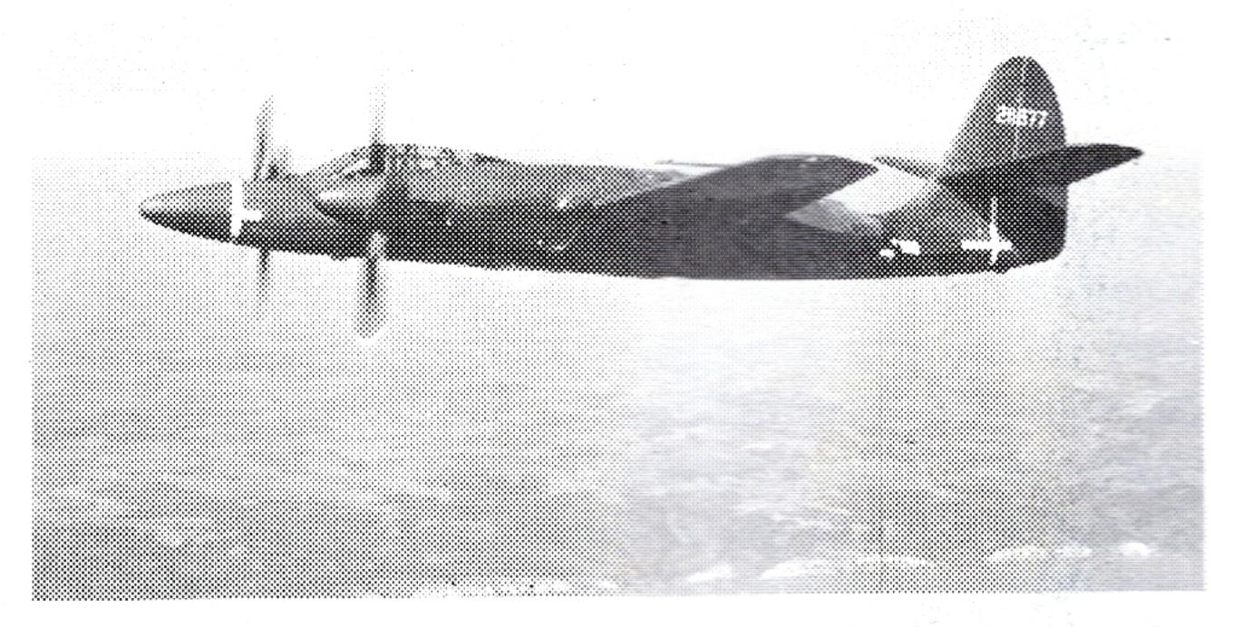
The XP-67 in flight over the Mississippi after cooling duct inlet and tailplane modifications.
