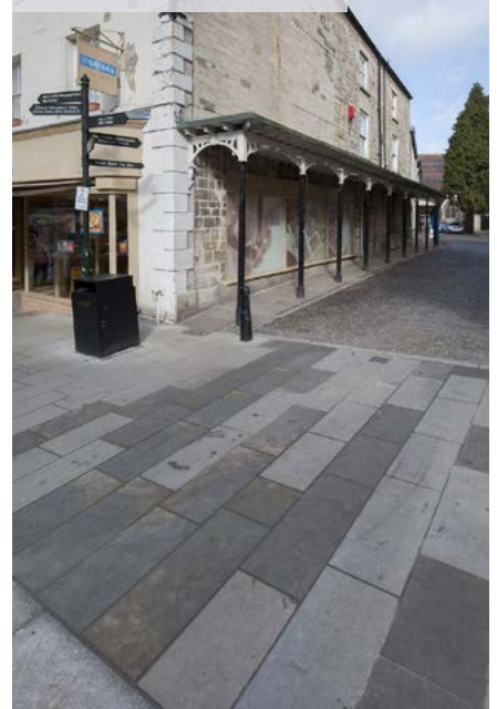
Larger Format Paving Is More Bedding Dependent
