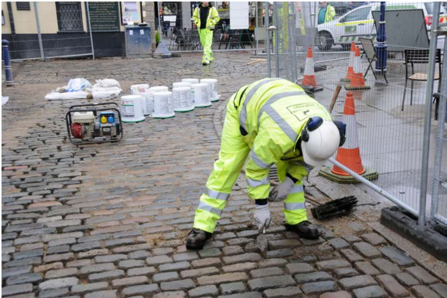
Larger Format Paving Is More Bedding Dependent
