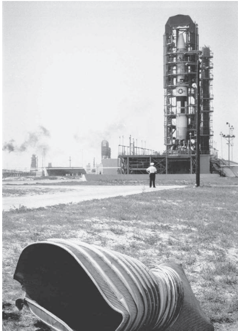
Figure 4.2. Titan II N-4 (60-6811) sits on Pad 16, Cape Canaveral, Florida, 27 June 1962, shortly after the first and only ground abort in the Titan II ICBM research and development program. A combustion instability at the Stage I Subassembly 2 injector cut the thrust chamber off. It came to rest several hundred feet from the flame deflector. N-4 had a new Stage I engine set installed within a month and was successfully launched on 25 July 1962. Courtesy of Robert Stahl.
