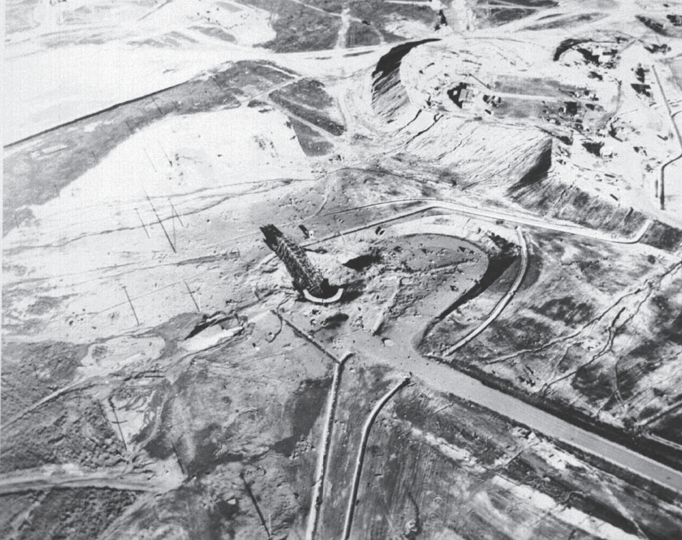
Figure 2.6. Aerial view of the aftermath of the 3 December 1960 explosion at the Operational Suitability Test Facility, Vandenberg AFB, California. The three operational training sites for Titan I can be seen in the upper right hand corner of the photograph. The large structure protruding out of the silo is the “crib” which supported the missile thrust mount and flame deflector. It was ejected straight up from the silo, cartwheeled 180 degrees, and slammed back down into the silo. Courtesy of Fred Epler.
