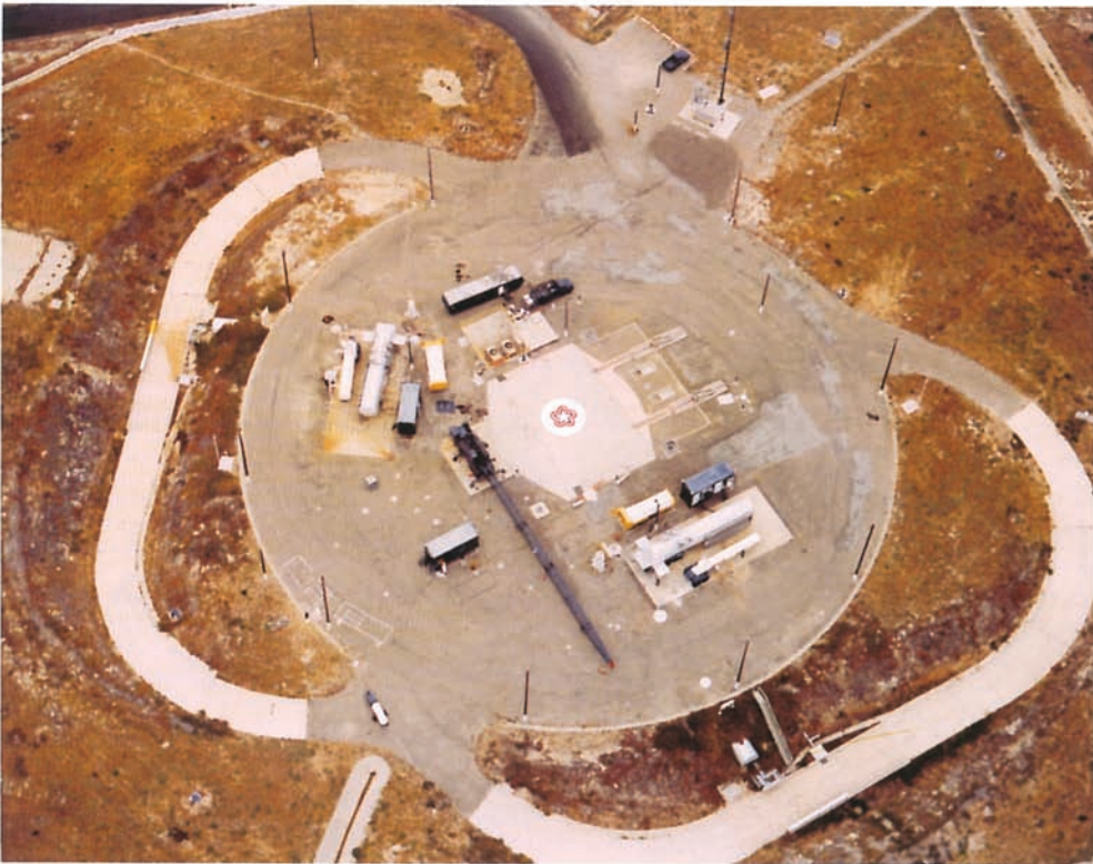
Figure CI.7. Launch Complex 395-C, Vandenberg AFB, California, during propellant transfer operations in preparation for the launch of Titan II B-17 (62-2771). The bicentennial emblem is clearly evident on the silo closure door. Initial plans were to launch B-17 on 4 July 1976, but range safety considerations required moving the launch date to 27 June 1976. Courtesy of Randy Welch.
