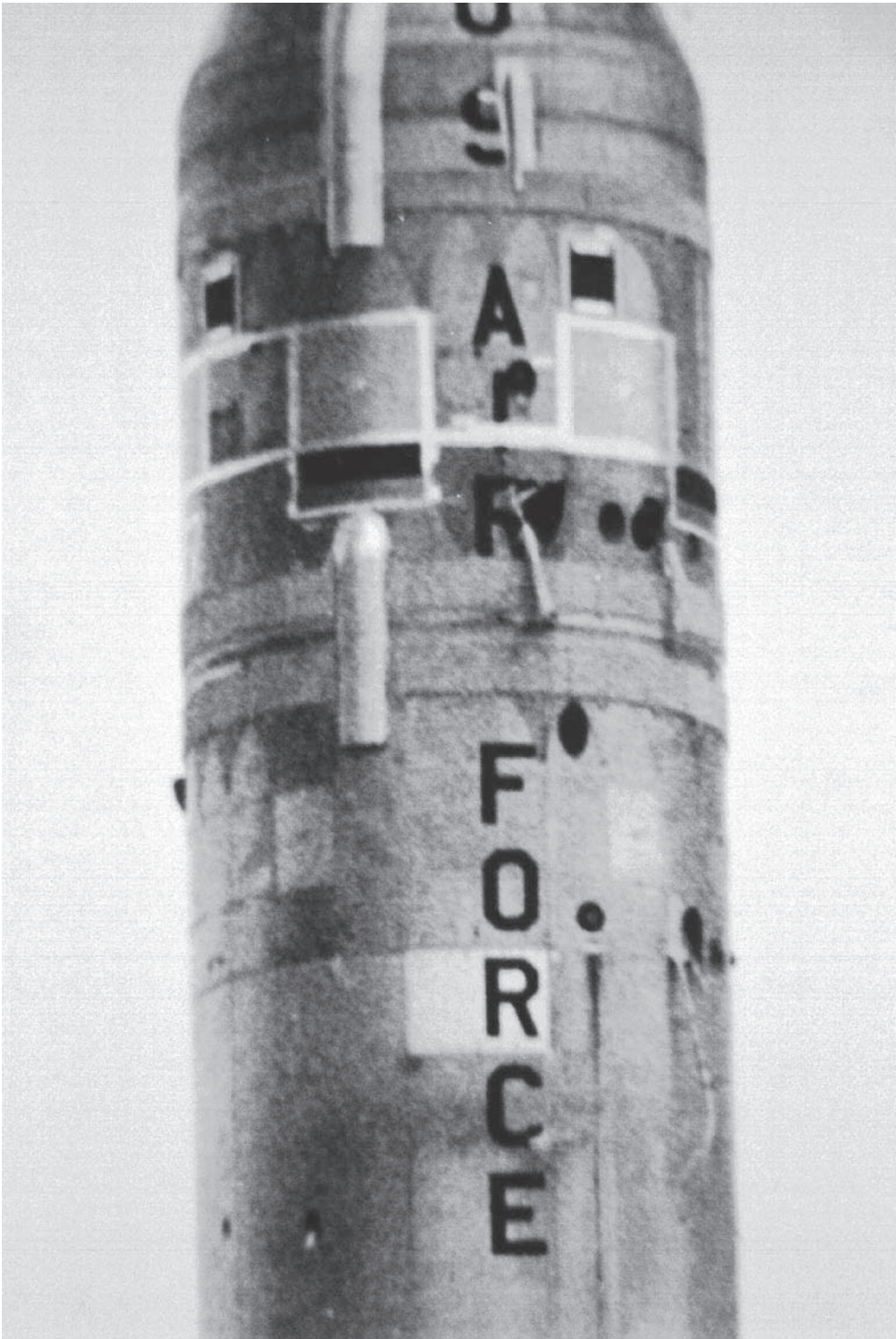
Figure 4.8c. Enlarged section of 4.8b showing the torn wiring hanging from the side of the missile. Courtesy of F. Charlie Radaz.
