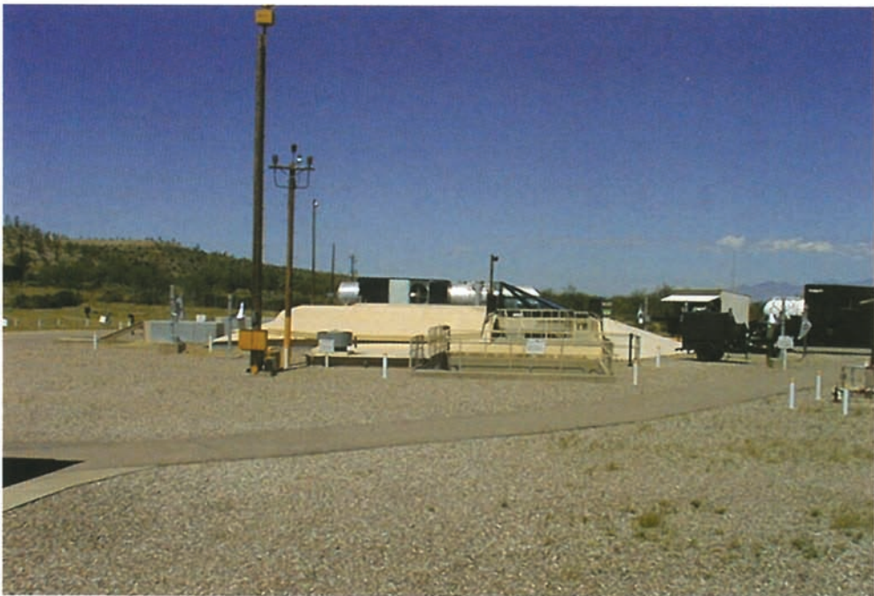
Figure CI.8. View looking north at the entrance to Launch Complex 571-7, the Titan Missile Museum National Historic Landmark. The structure in the center of the photograph is the silo closure door with the environmental cover over the launch duct. Courtesy of the Titan Missile Museum National Historic Landmark Archives, Sahuarita, Arizona.
