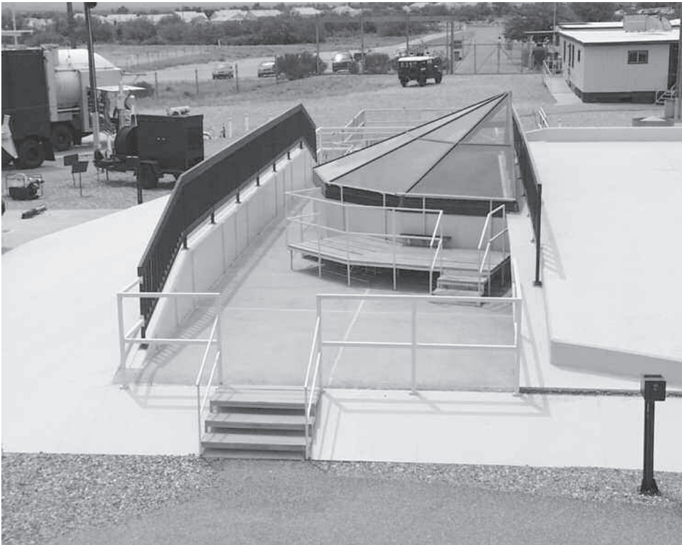
Figure EP.5. View of the launch duct observation window at Launch Complex 571-7, the Titan Missile Museum National Historic Landmark, Sahuarita, Arizona. The exhaust ducts have a covering of concrete to facilitate access to the viewing area. Courtesy of the Titan Missile Museum National Historic Landmark Archives, Sahuarita, Arizona.
