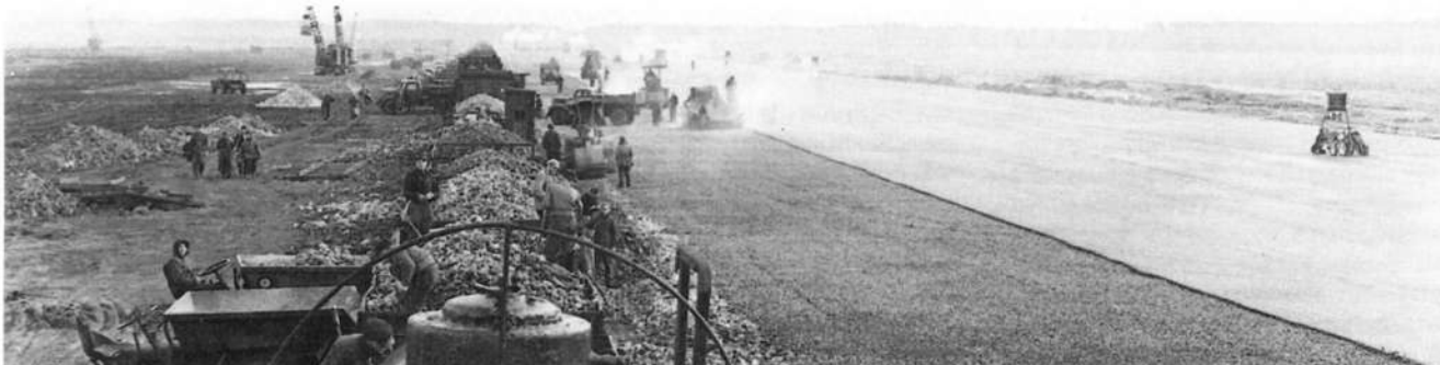
High intensity operations demanded much airfield maintenance. German labourers are shown widening a landing strip. via Bruce Robertson
