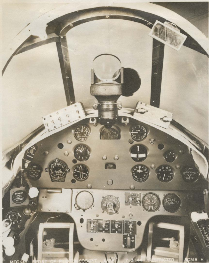
MOCKUP FRONT OF PILOT'S COCKPIT XFB 7-3-44 RESTRICTED 0318-B
