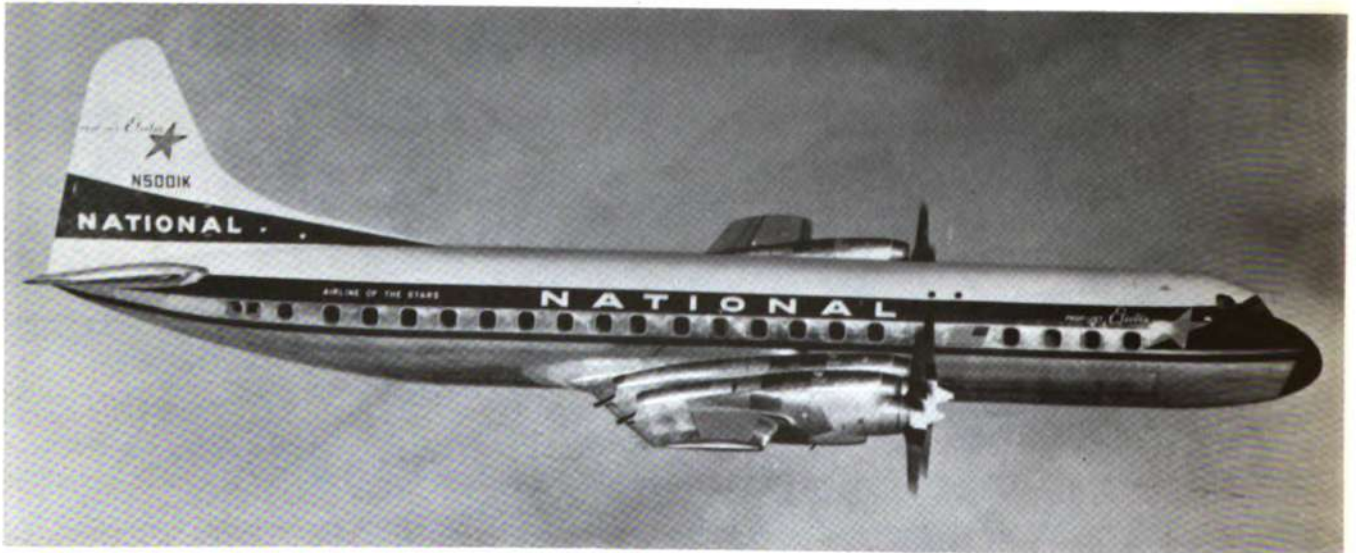
The Lockheed ELECTRA is a four-engine, turboprop airliner.
