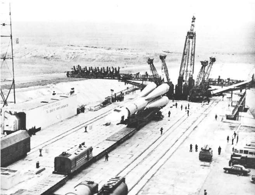
An A-2 moves slowly back on to the support pedestal from where it will be launched. Note the erector on which the launch vehicle rests during transport.
