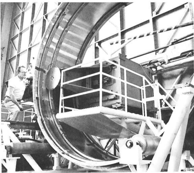
The Atlas missile was assembled from cylindrical skin sections here being seam-welded from flat sheets of alloy.
