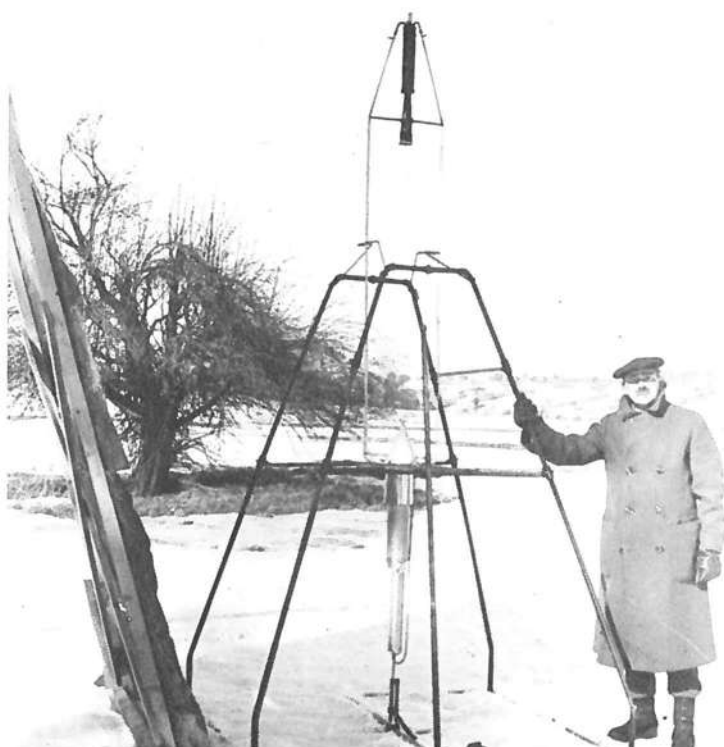
This historic scene records the actual liquid propellant rocket that → became the first of its kind to fly on 16 March 1926, at Auburn, Massachusetts. Robert Goddard, the 'father of the rocket', is seen shortly before it took off for a flight lasting 2½ sec.
