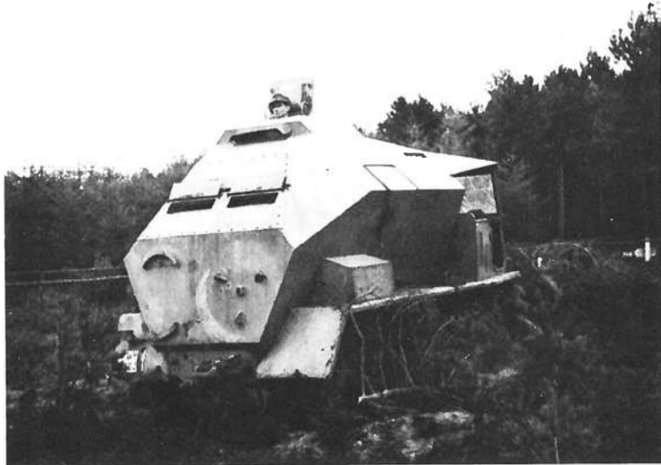
The Firing Control Vehicle from which final countdown and launch preparations were conducted before ignition of the V-2 propulsion system.
