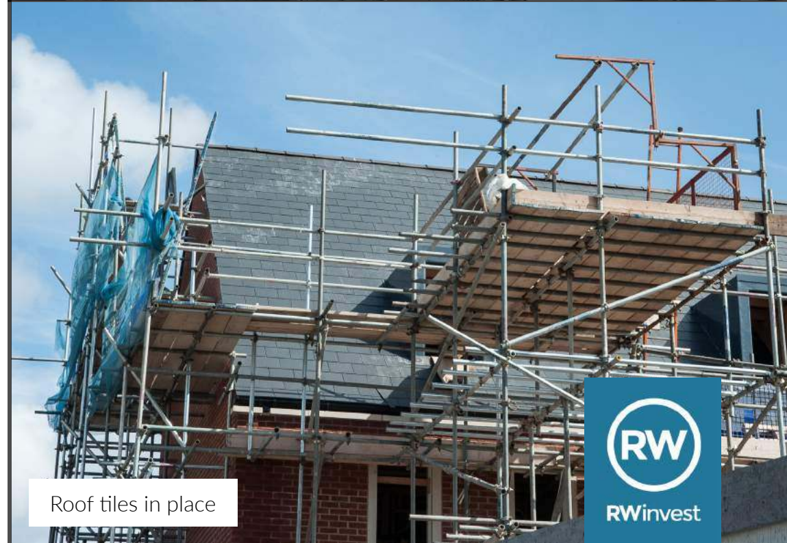
Roof timbers being installed
