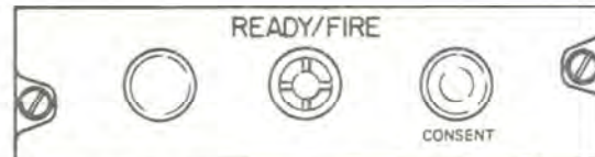
N READY/FIRE CONTROL PANEL
