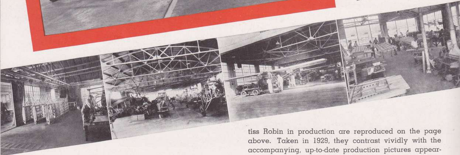
Above, Curtiss-St. Louis factory scenes of 1929. Note the production line which Curtiss introduced to the aviation industry when manufacturing the famous Robins. Many interesting features catch the eye in these pictures. For instance, the modern type illumination in the Final Assembly Department shown at left, or directly underneath, the view of the panel department which shows several woodworkers — artisans no longer used in aircraft production. Second from left below, one of the first, if not the first, ship produced by Curtiss on Lambert Field.
