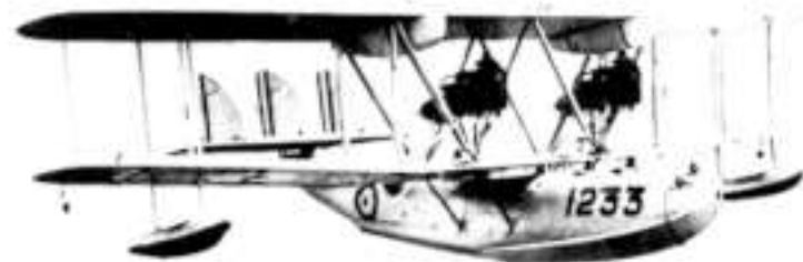
The first flying boat of post-war design to enter RAF service was the Supermarine Southampton, one of R J Mitchell's first military aircraft designs. About 20 Southamptons had wooden hulls (below) but most were converted to metal-hulled Mk IIs (above) and about 50 more were built as such.
