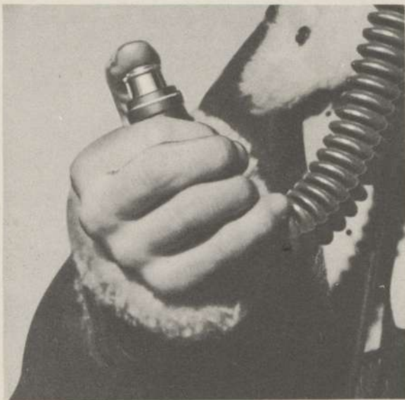
Gentle suction test for mask fit.
