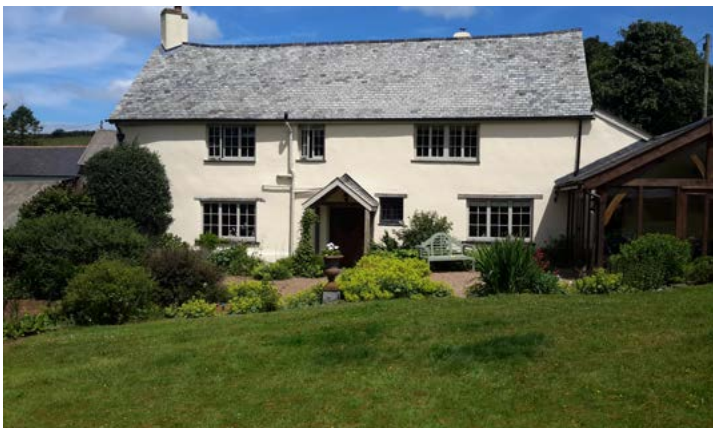
External walls are painted with the Sandstone shade of Ecopro Silicate Masonry Paint, providing a long lasting alternative to limewash.
