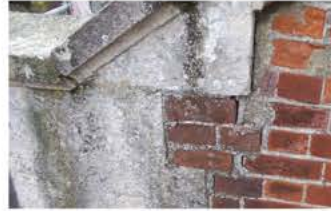
Failing Brickwork
