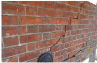
Cracking Wall/Brickwork
