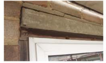
Failing Lintel
