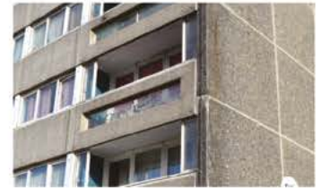
Large Panel System building (LPS Blocks)
